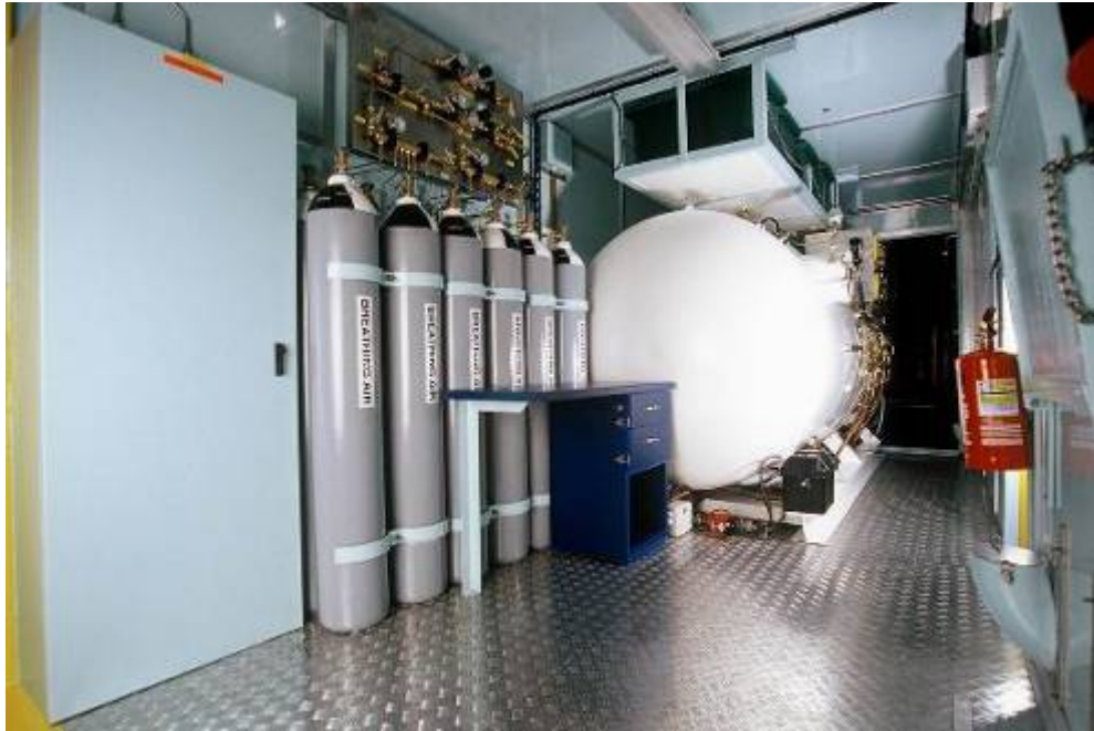
Figure 2: Typical Chamber with 12 cylinder bank and insulated container
